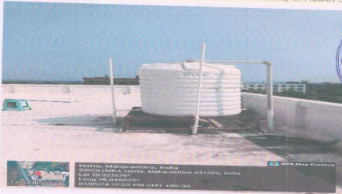
Water Harvesting tank (Capacity-1000L)
